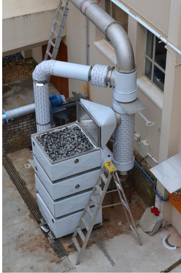
Figure D-1: High temperature test facility showing test section with top plenum chamber removed
