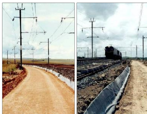
Figure 2.8: Geotextile as a filter medium under and next to railway (Kaytech)
