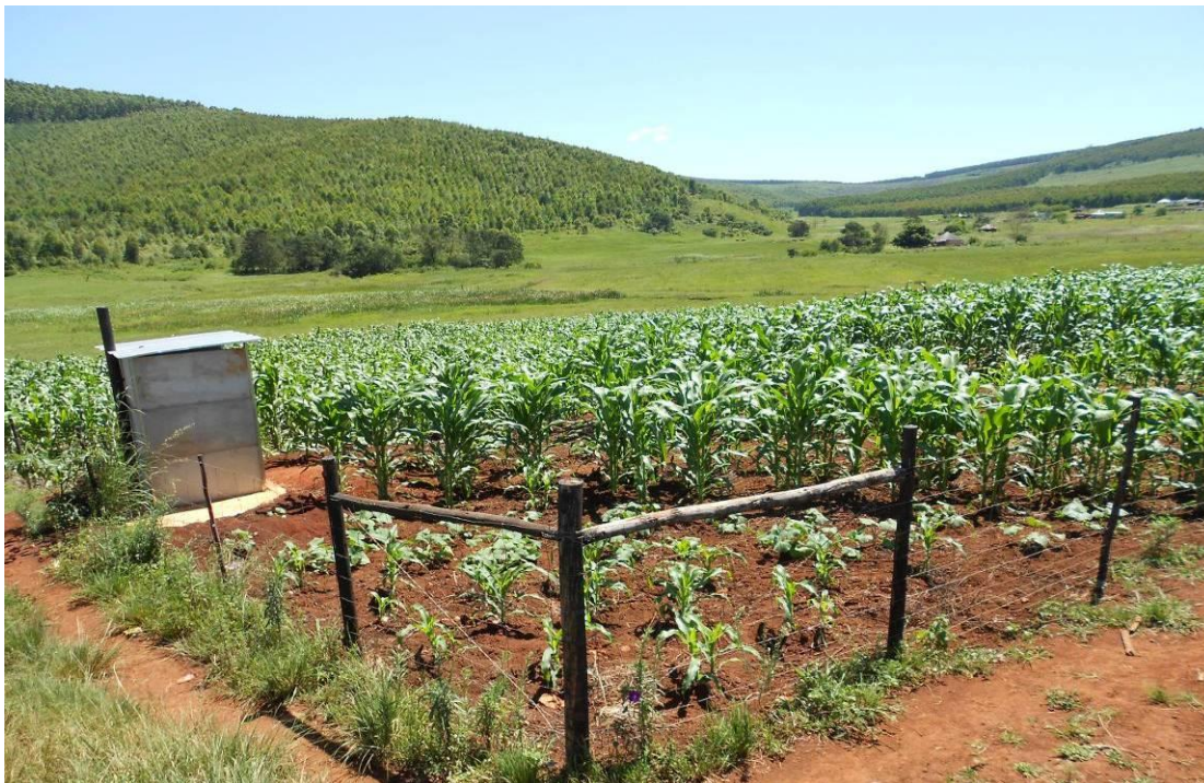
Figure 8: Fence construction, showing 'Veldspan' fence, and corner structure
