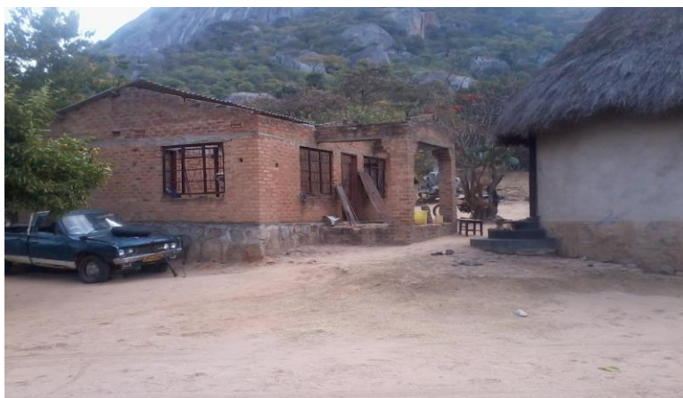
Figure 7d: A house which had been put on hold for years and is now being finished
