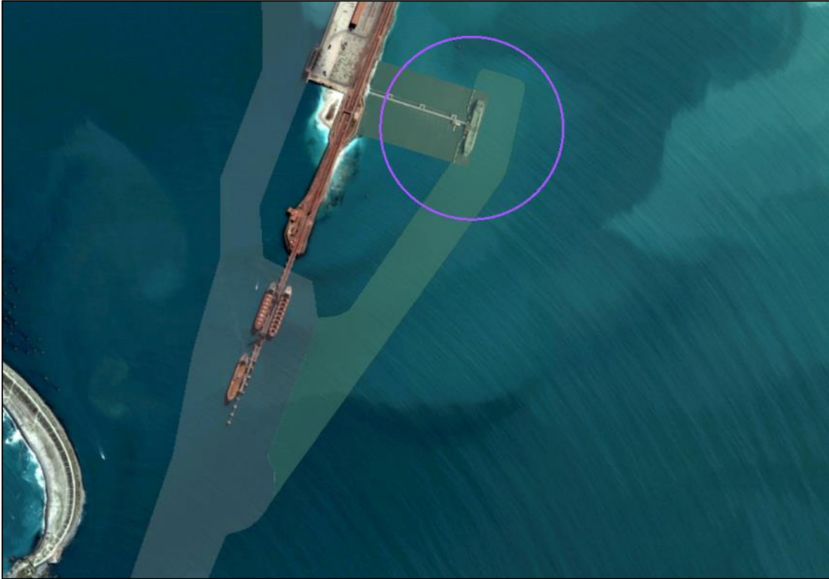
Figure 9-13 Navigational zones nearby Site 3 - Big Bay: Causeway
