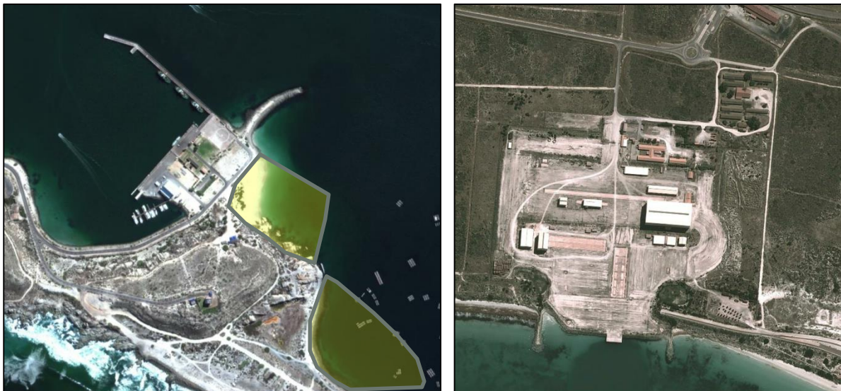
Figure 9-29 Small craft quay in Hoedjiespunt (l) and the Mossgas quay (r)
