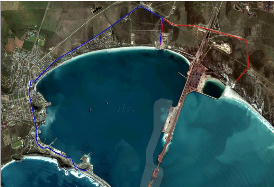
Figure 9-30 Road infrastructure from Mossgas quay to Hoedjiespunt (blue, on left) and to CCGT site (red, on right)
