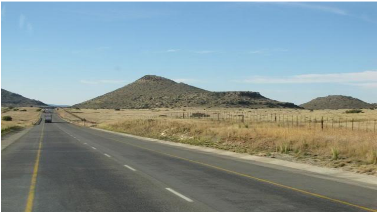
Figure 2. 4: Typical two-lane two-way highways in South Africa (Google earth)
