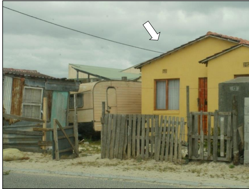
Figure 6.2. Informal shacks attached to a main house in Makhaza, Cape Town. The arrow indicates the original house (Massey 2011)
