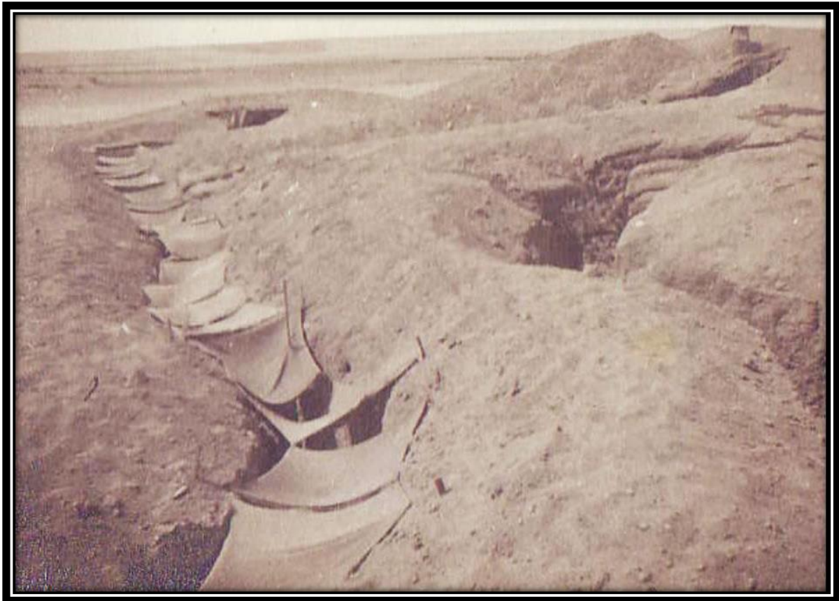
Figure 4.2: C Company trench system at Mersa Matruh. 396
