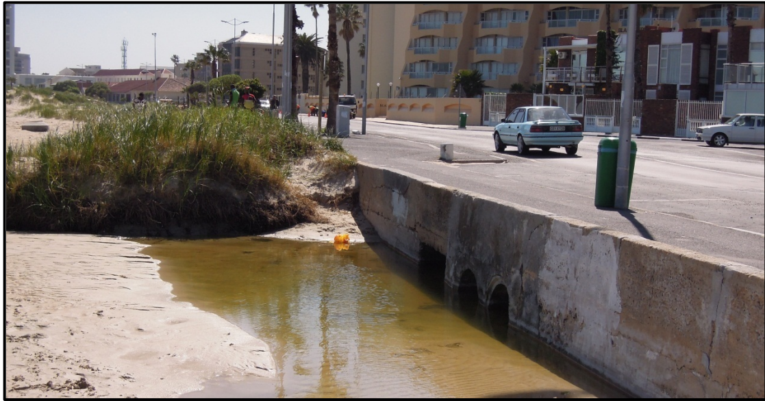
Figure 29: Sand dune in front of a vertical wall, near location H (05/09/2012)
