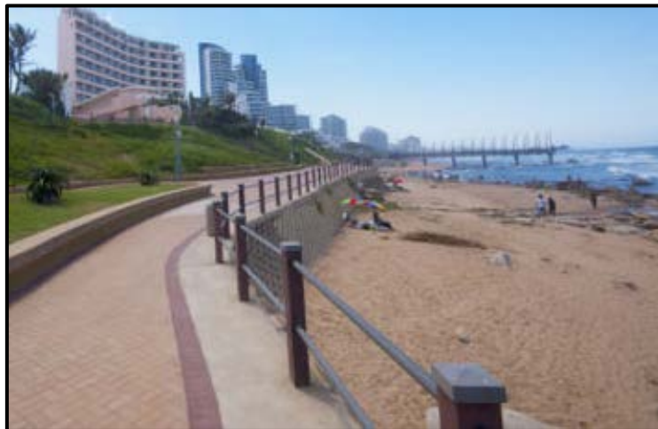
Figure 17: Sloped seawall at Durban, KwaZulu-Natal (Steel, 2011)
