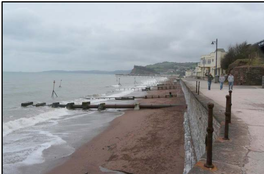
Figure 22: Vertical wall at Teignmouth, Devon (Gayton, 2010)
