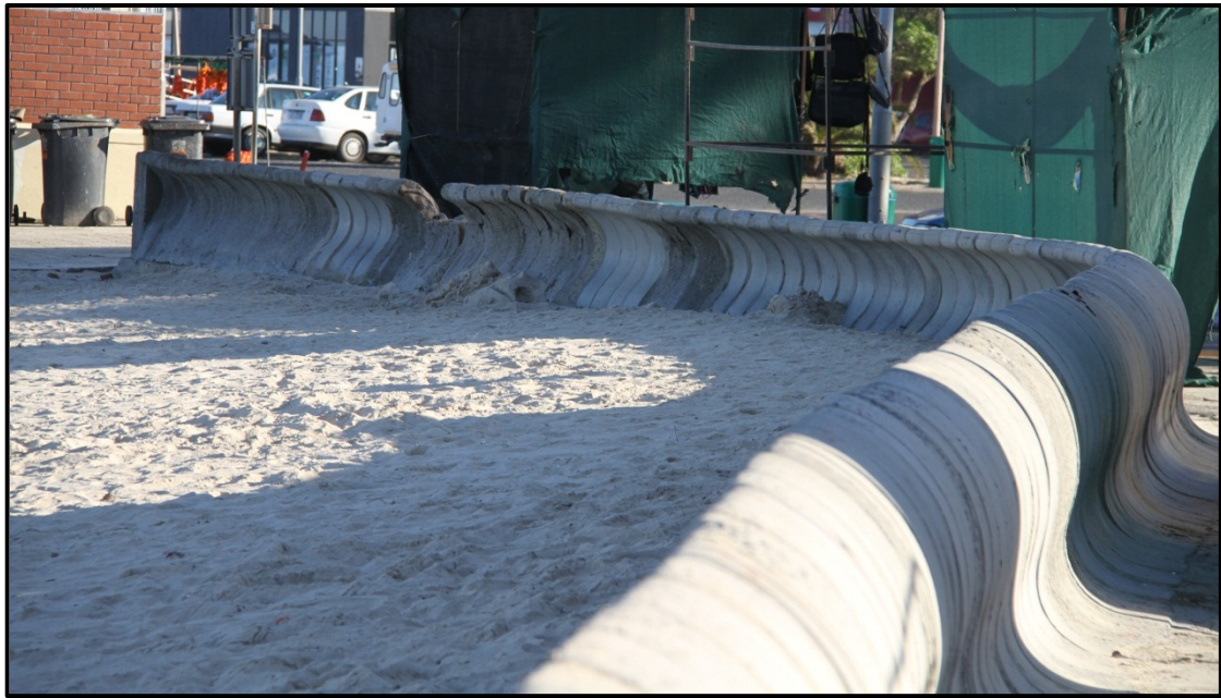
Figure 32: Recurve wall along the parking area at location F (05/09/2012)
