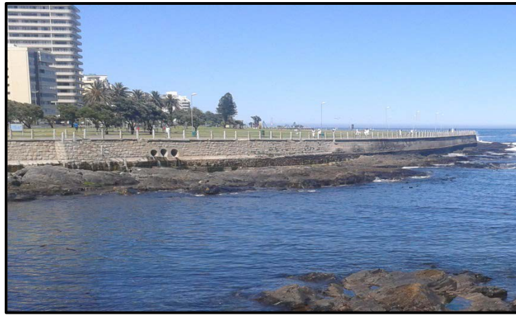
Figure 16: Seawall with parapet at Cape Town, Western Cape (Cape Town Collectables, 2012)
