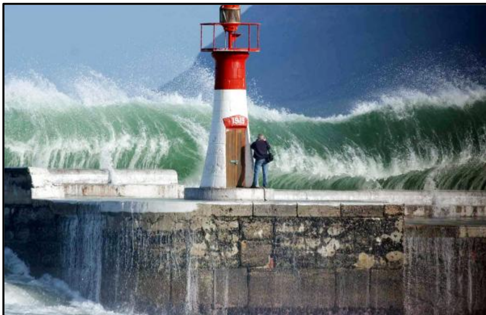
Figure 3: Wave overtopping at Kalk Bay harbour during August 2005 (Hunter, 2005)
