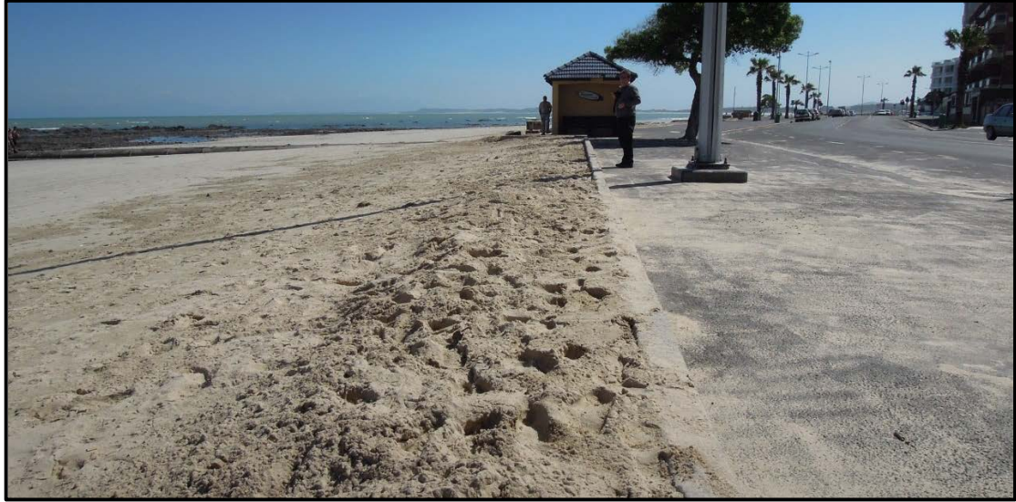
Figure 30: Vertical wall with sand built up to the top of the wall at location E (05/09/2012)
