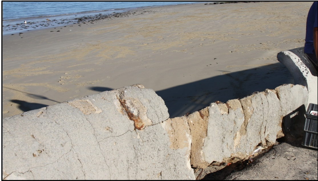
Figure 33: Damaged recurve wall at location F (05/09/2012)
