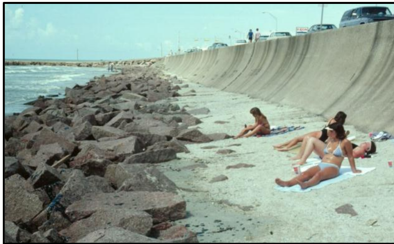
Figure 19: Rock revetment and seawall at Galveston, Texas (Marine Insight, 2012)
