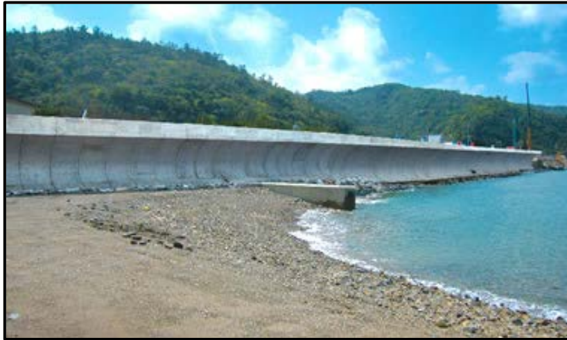
Figure 18: Flaring seawall at Kunigami, Okinawa (Kobelco, 2012)
