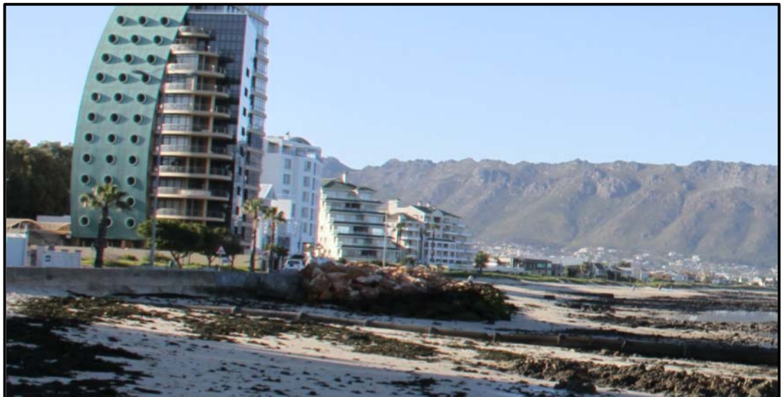
Figure 36: Composite vertical wall at location I, looking east (19/07/2012)
