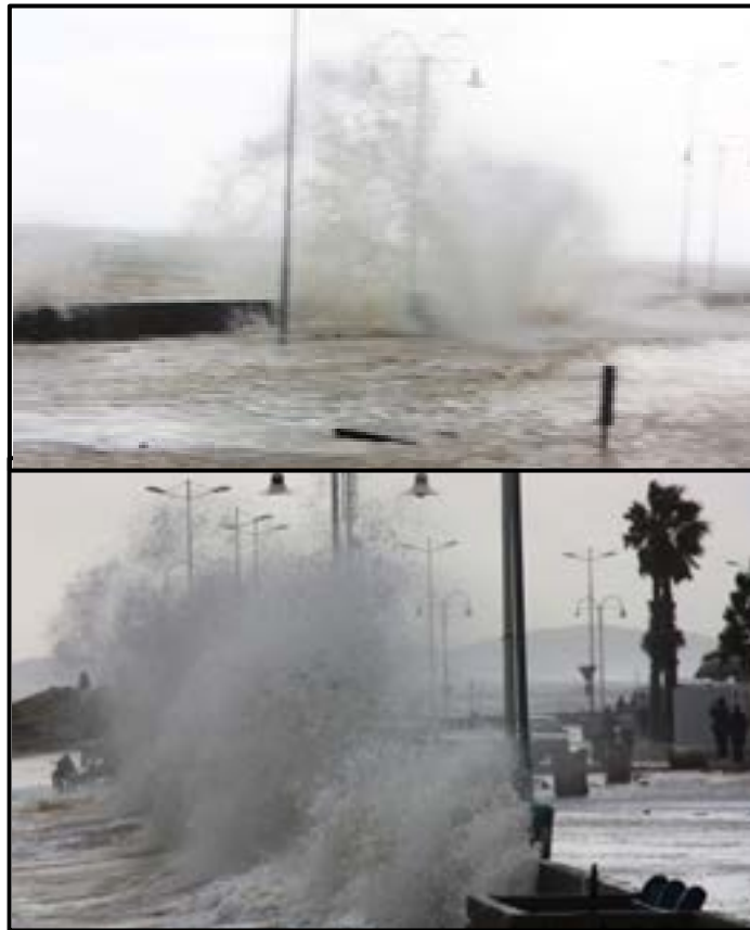
Figure 1: Overtopping during August 2008 (Cape Town Gazette, 2008)
