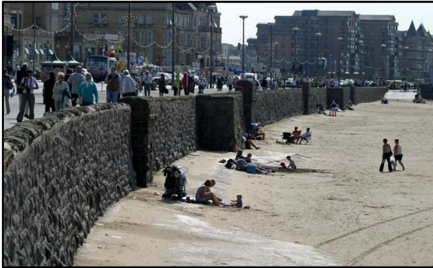
Figure 21: Vertical seawall at Weston-super-Mare, Somerset (The Telegraph, 2012)
