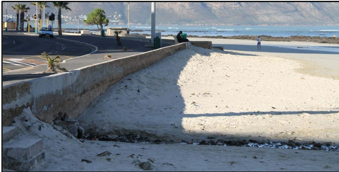
Figure 31: Vertical wall with stormwater outlet near location H (05/09/2012)
