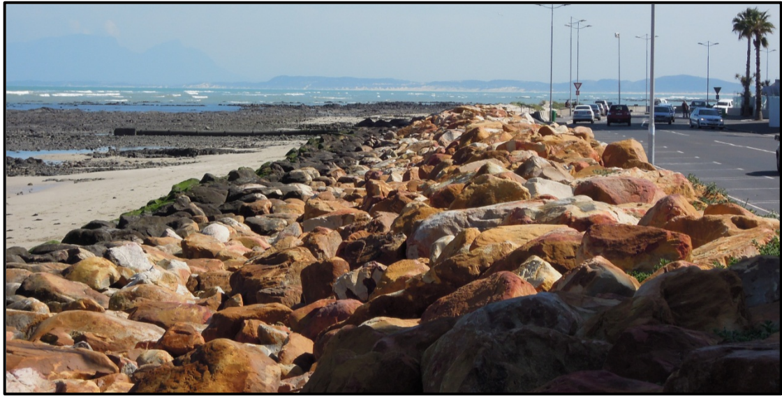
Figure 35: Composite vertical wall at location I, looking west (19/07/2012)
