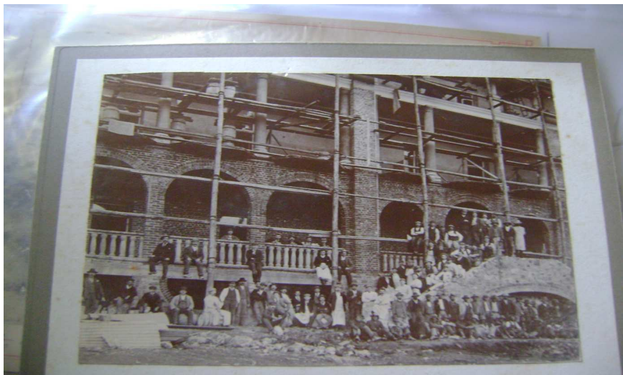
Construction at the Caledon Sanatorium, n/d (Photo without reference, Caledon Museum).
