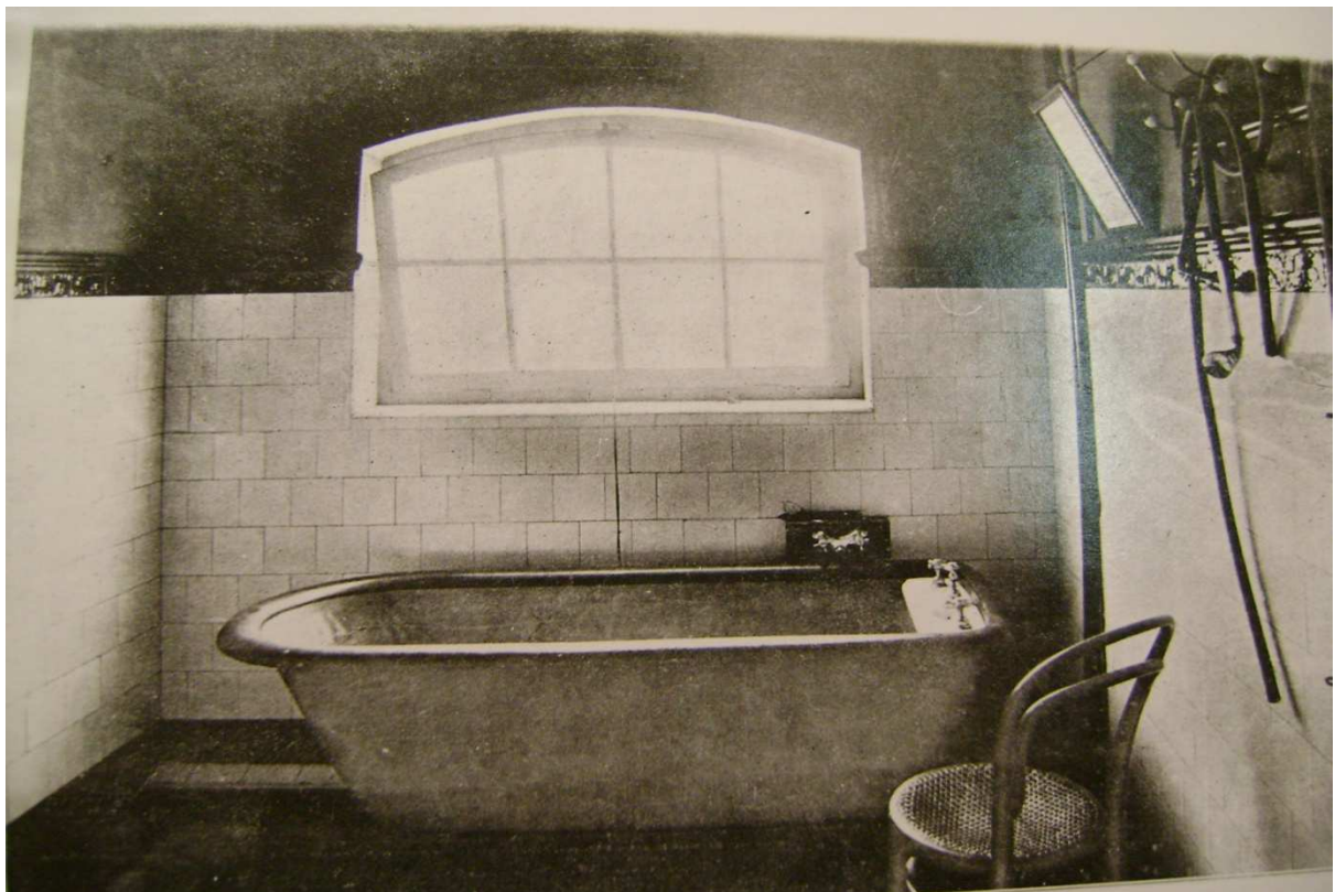
A bathroom at the Caledon Sanatorium, n/d (Jeffreys Collection, J7449).
