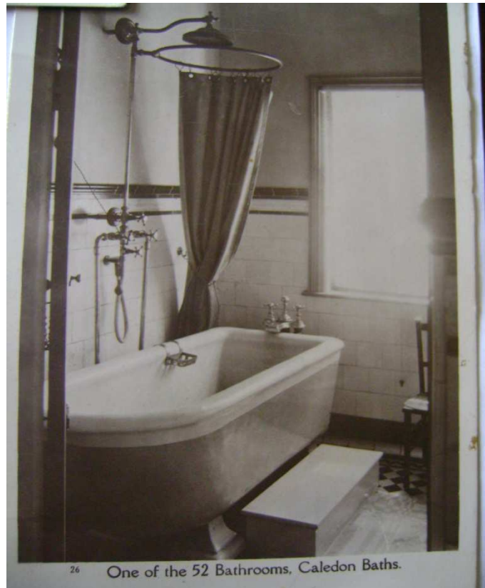
One of the Bathrooms at the Caledon Sanatorium, n/d (Photo without reference, Caledon Museum)
