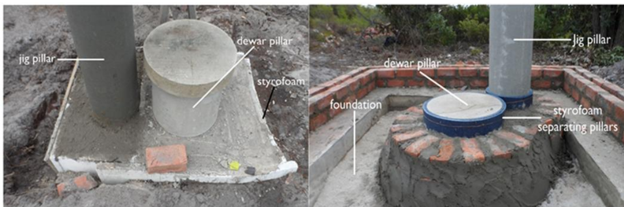
Figure 3.12: Dewar and jig pillars of the Hermanus SQUID system during the construction phase of the non-magnetic hut. The Styrofoam was laid in order to decouple the pillars from the floor and walls of the building as well as provide some damping of mechanical vibrations in the ground.
