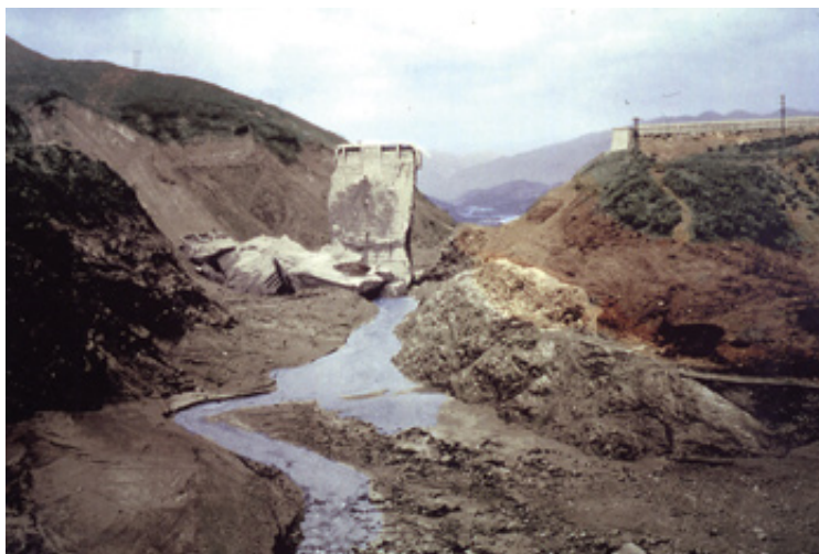
Figure 2.4: Photo of failed St. Francis Dam, California (Cervin, 2008)
