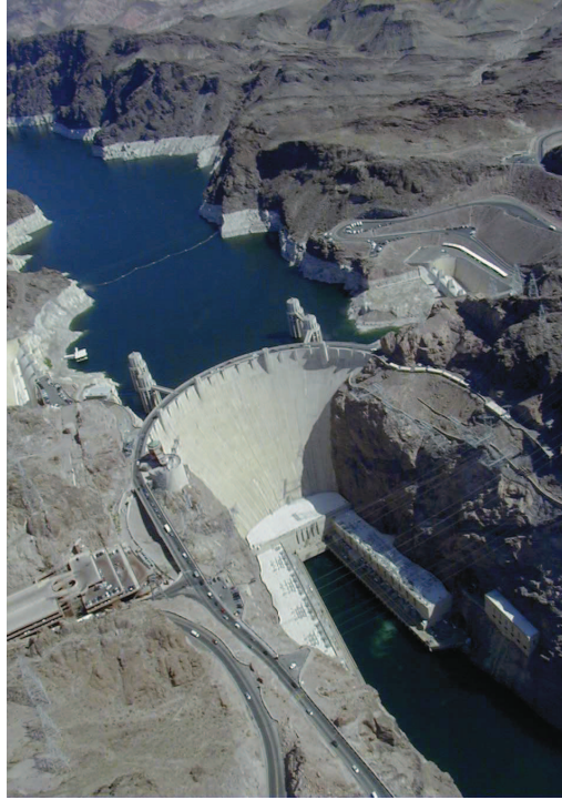
Figure 2.1: Hoover dam constructed by the Bureau of Reclamation in the USA (WePhotographer, 2004)
