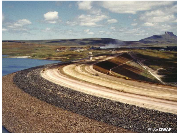
Figure 2.2: Example of an embankment dam, Sterkfontein Dam in South Africa (DWA, 2012)
