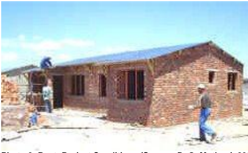
Photo 2: Post- Project Conditions (Source: D. G. Mothusi, 2001)
