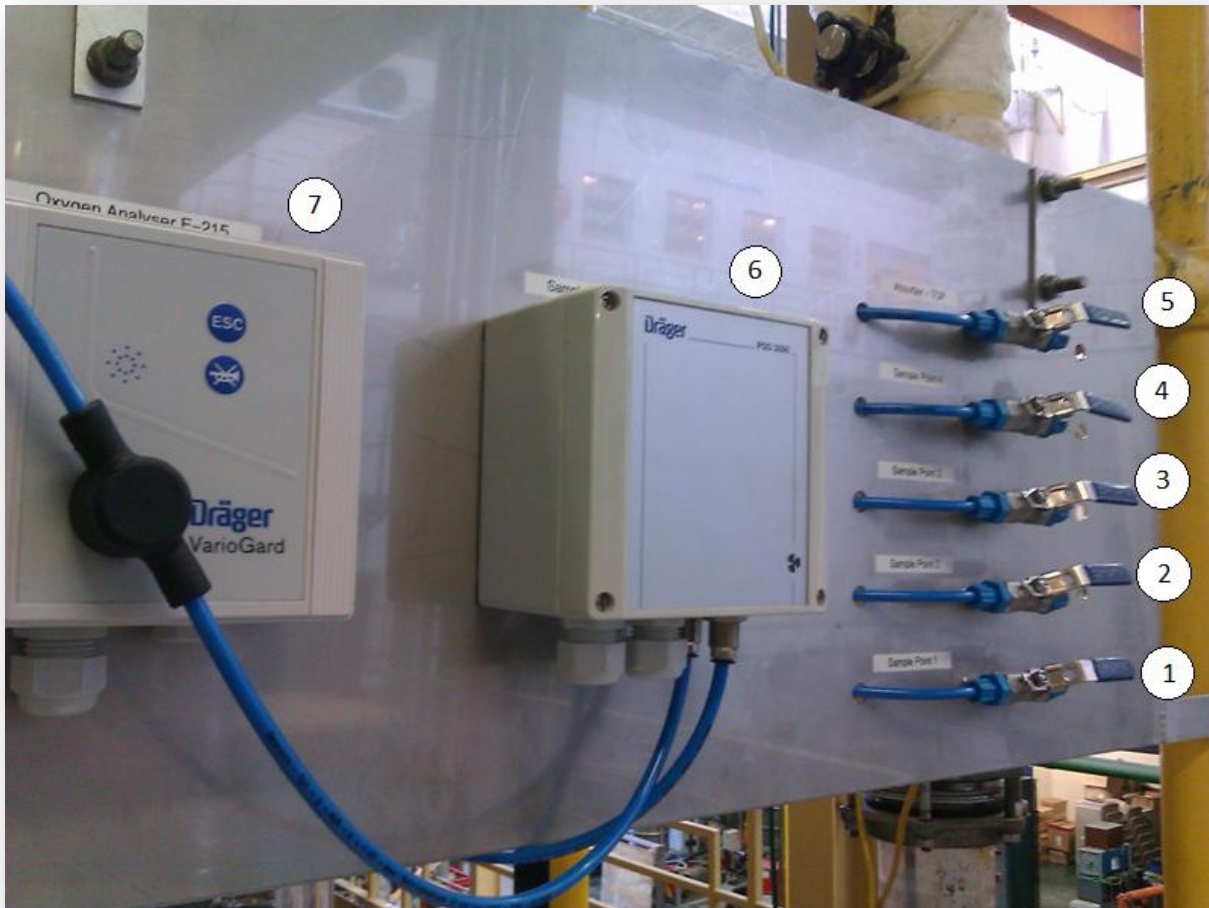
FIGURE 25 GAS SAMPLING VALVE MANIFOLD SETUP
