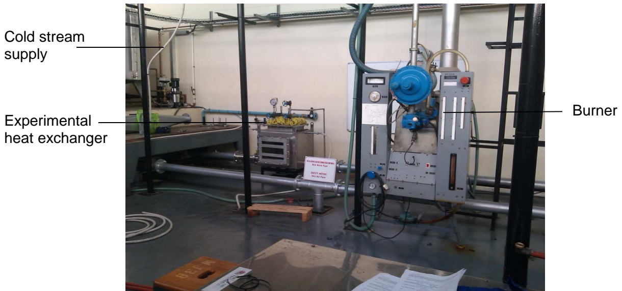
Figure 4.4: Photograph of the heat pipe heat exchanger and hot gas supply burner
