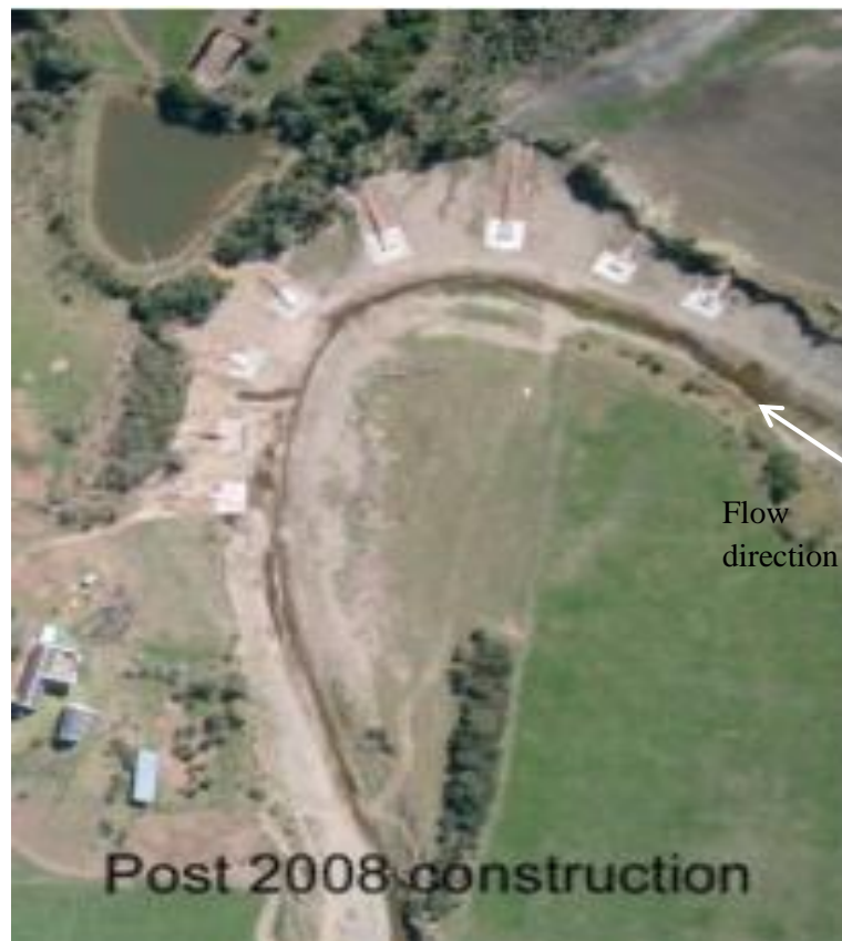
Figure 12: Tradouw project after construction in 2008
