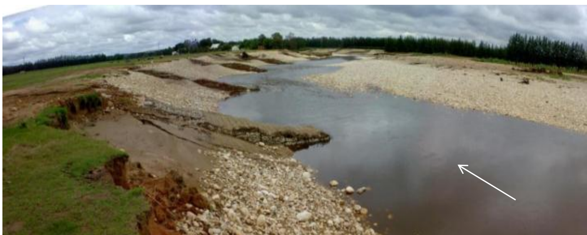
Figure 135: Mullersrus after 2008 flood
