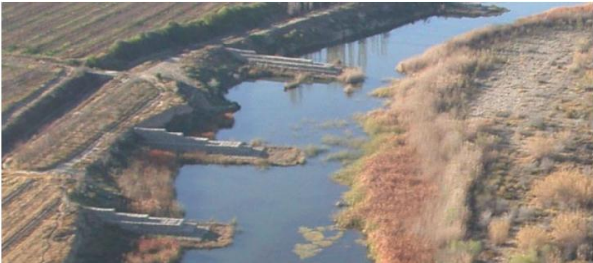
Figure 2: Groyne protection around a bend in the Gamka River, Calitzdorp (King, 2009)
