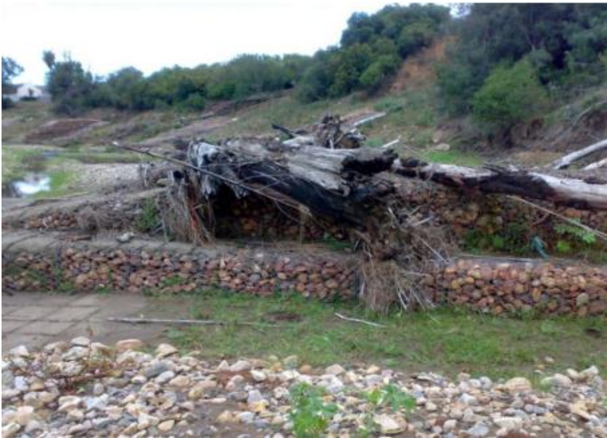
Figure 131: Debris found on groynes after flood (Tradouw)
