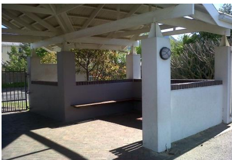
Newly constructed meeting zone at school PP
