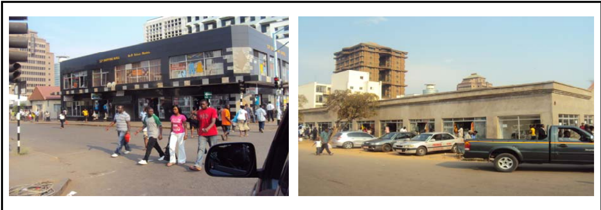
Partitioned buildings to accommodate IEEs within the CBDs during the 2000s (Harare)
