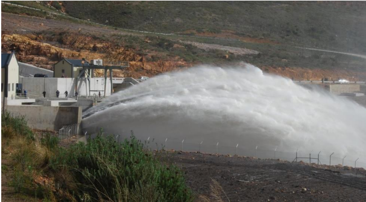
Photograph 14: Commissioning test (2008) (close-up)
