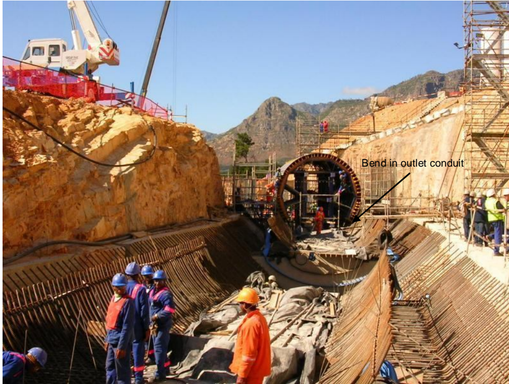
Photograph 12: Outlet conduit being built
