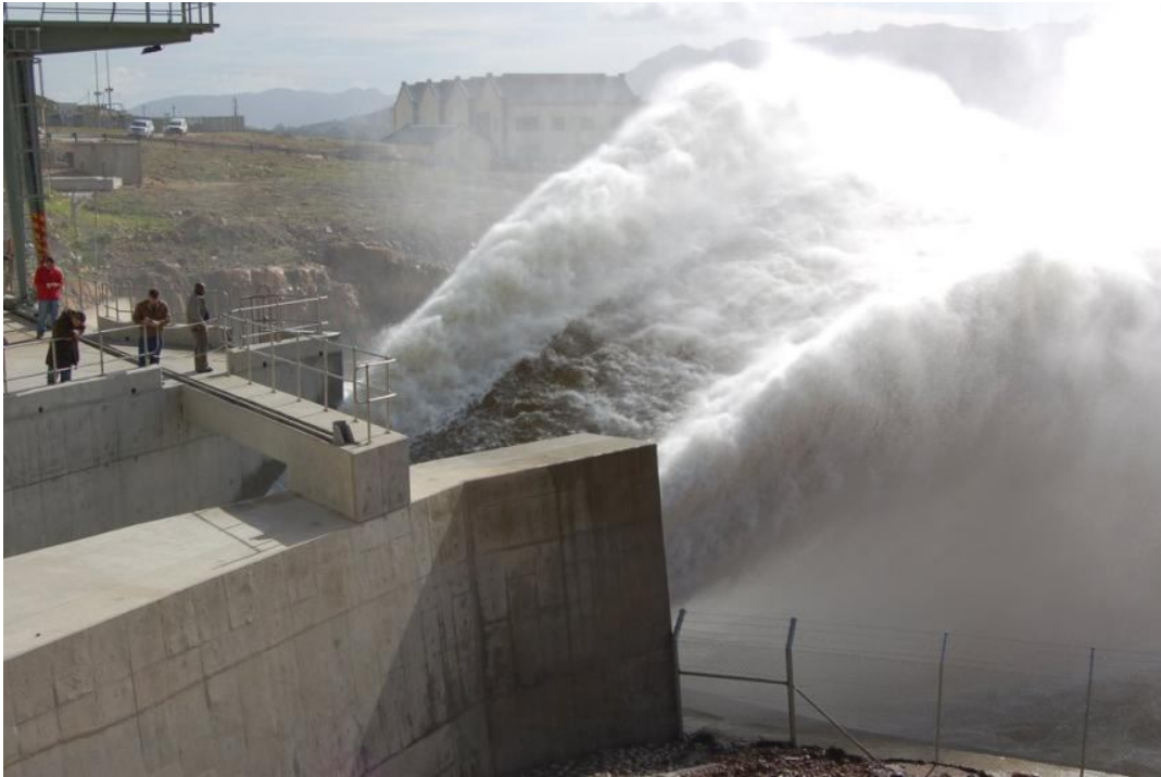
Photograph 17: Top view of flood release during commissioning test (2008)
