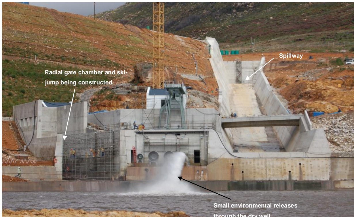
Photograph 18: Berg River Dam outlet structures during construction phase
