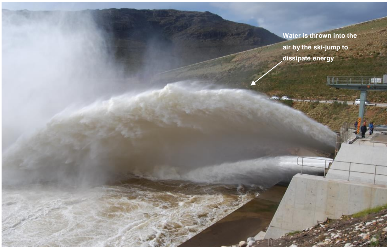
Photograph 15: Commissioning test (close-up)
