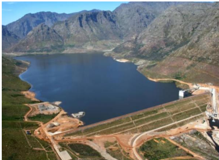
Figure 1.2: Berg River Dam
