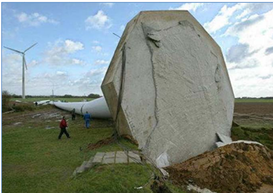
Figure 29: Failed wind turbine foundation design
