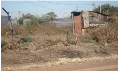
A single pit latrine on a large stand in Evaton
