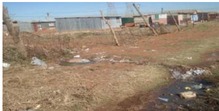
Sewerage blockage in Hamilton Road, Evaton
