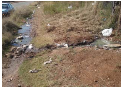
Sewage spillage from the manhole along one of the streets
