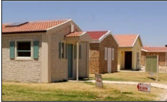
Photo 5: A typical gap unit built by the city of Cape Town Source: http://www.capetown.gov.za/en/GapHousing
