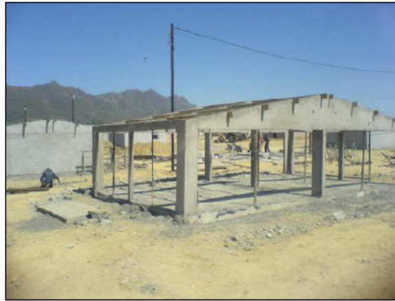
Photo 1: Swartland's concrete mould for RDP units Source: Swartland Municipality (2007: 8)
