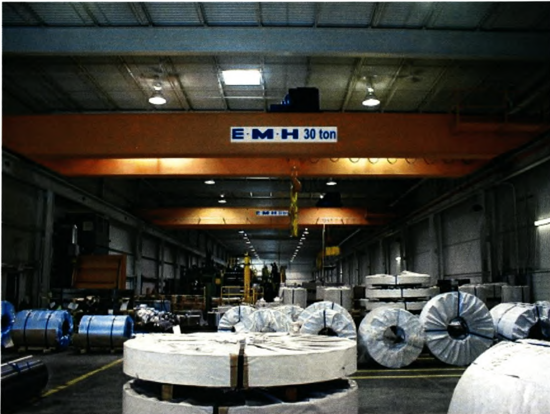
Fig. 1.1 Overhead crane in an industrial building
