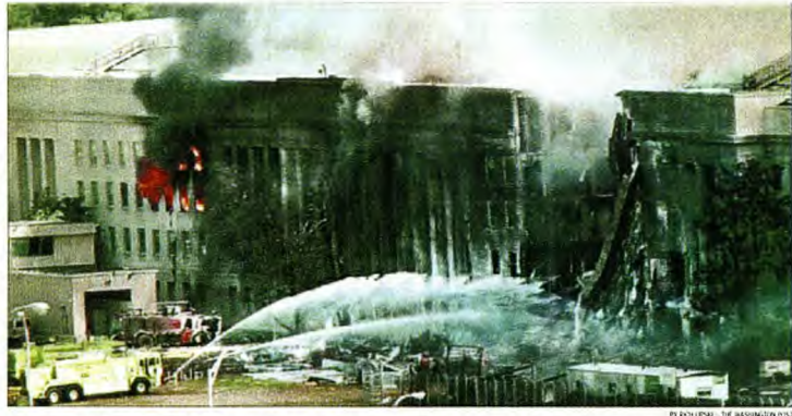
Firefighters battle blazes at the Pentagon, which was hit by a plane that had been hijacked after taking off from Dulles International Airport.
