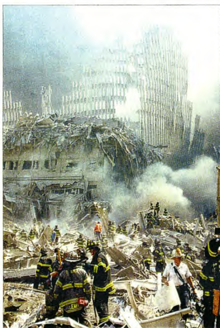
A shell of what was once part of twin 110-story towers at the World Trade Center rises above the rubble, leaving a huge gap in the New York skyline.
