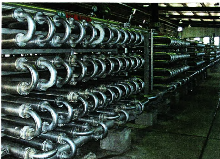
Figure 2.2. UF membrane plant in the Mondi Kraft paper mill at Piet Retief.
