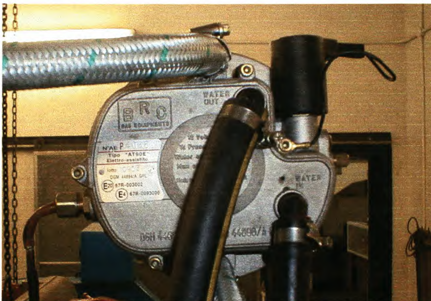
Figure 3.6 A LPG evaporator / regulator
