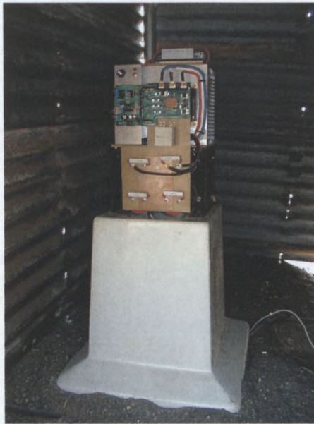
Fig. 67: 32 kVA single- to three-phase converter installed in stubby kiosk
