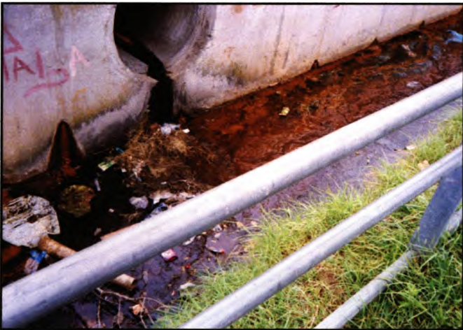
Fig. 4.2.3 They exit the stormwater drain at this point.
