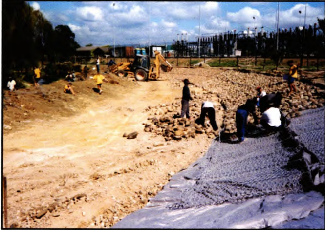
Fig. 4.1.5 The Council widening the banks of the river in preparation for the fifty year flood.
