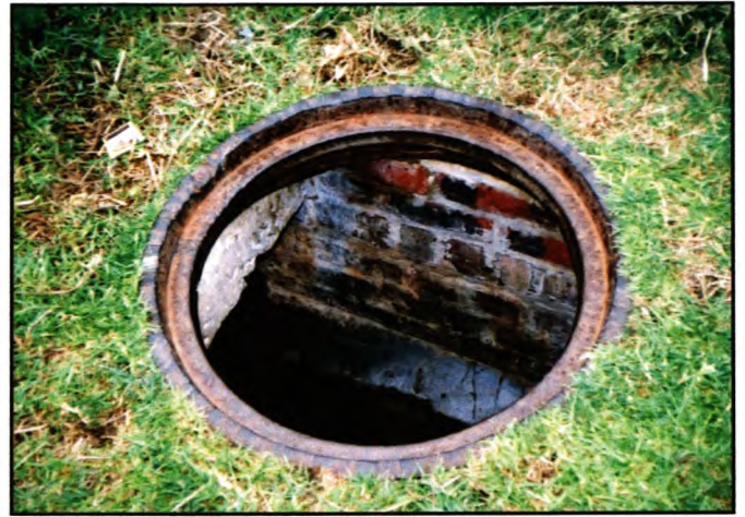
Fig. 4.2.2 Children climb into these stormwater drains for fun.
