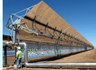
Nevada SolarOne - commissioned in 2007
