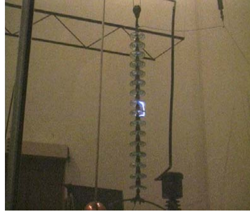
Figure 3.13: Local flashover across the two clean discs in the middle
