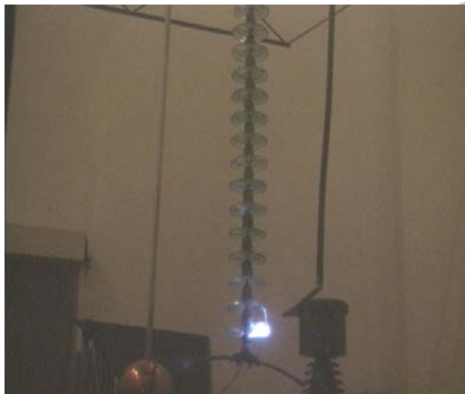
Figure 3.14: Local flashover across the two clean discs at the live end.
