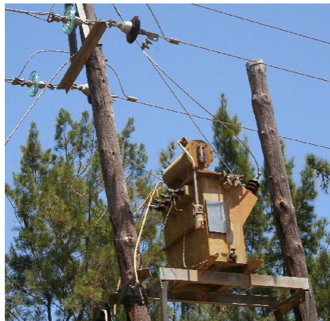
Figure 2.1: 50 kVA three phase pole-mounted distribution transformer
