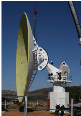
(a) The KAT during construction
