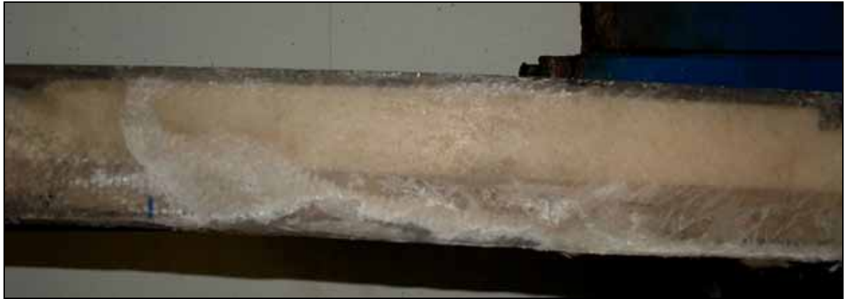
Figure 57: Delamination in composite beam
