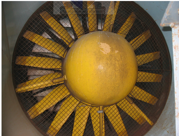
Figure C1.7: 2.7 m Diameter Suction Fan
