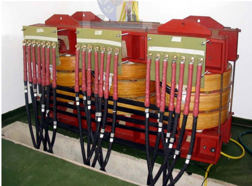
Figure 2.15 The Injection transformer
