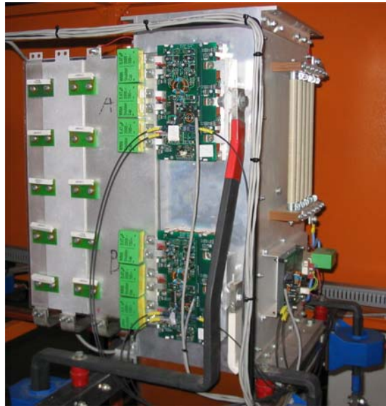
Figure 2.12 One of the seven three-phase full bridge inverters
