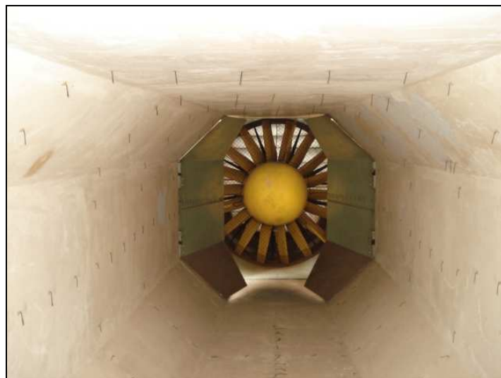
Figure 2.1: The suction fan and control gates
