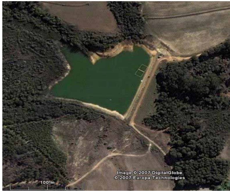
Figure 2.2: Aerial view of John Smith Dam at Rustenburg Wine Estate (Production site 2)
