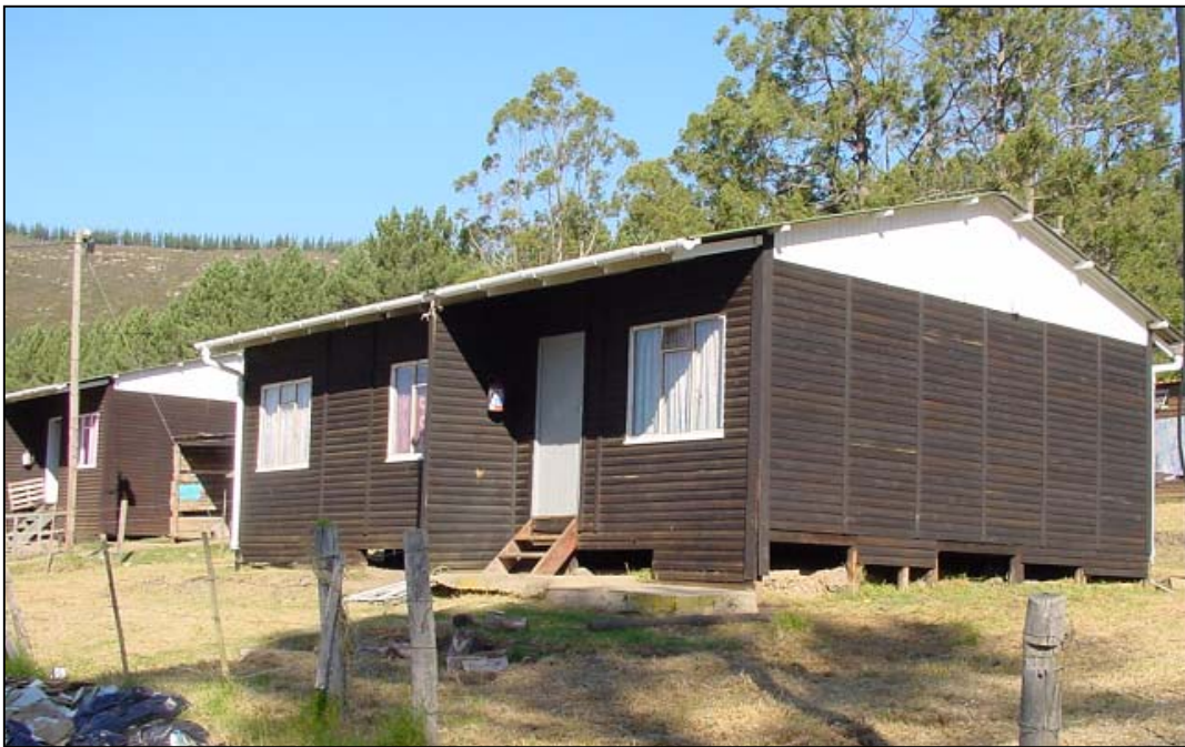
Figure 4.4 Housing in Sonskyn.
