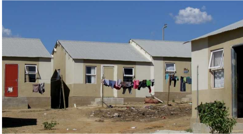
Figure 6: Completed semi-detached 40 m 2 house
