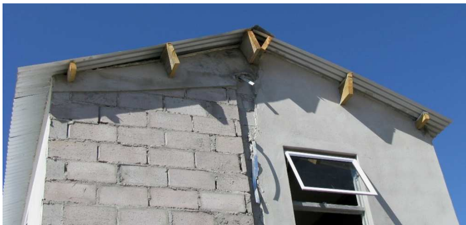
Figure 7: Typical roof construction of the conventional design
