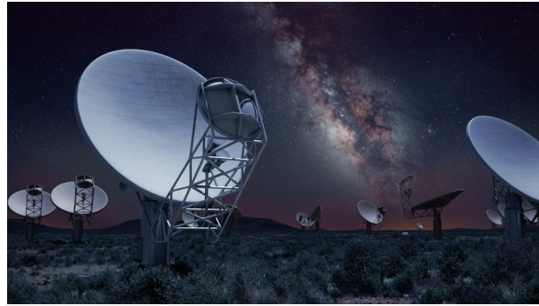
Figure 1.1: Prototype of a dual offset Gregorian dual reflector antenna for MeerKAT [3]
