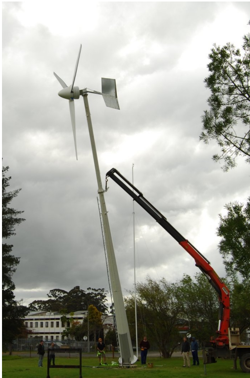
(a) Raising the 15 kW SS-PMG WECS and tubular tower on a pivoting base. The extension segment allows for a hub height of 18 m
