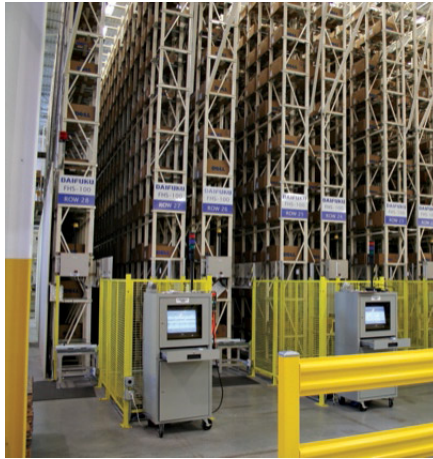
(a) A photograph of the control station for a single aisle in a AS/RS. Source: [8].
