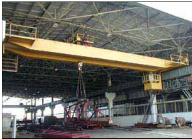
Figure 2.25: Example of a crane that is both outdoor and covered. The roof system stops, but the runways continue.
