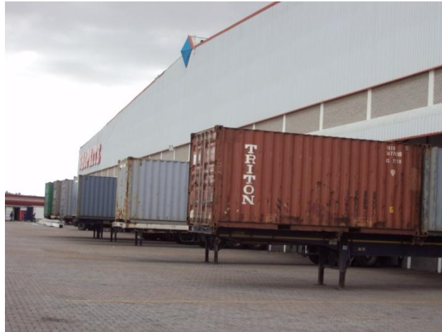
Figure 23: Container receiving bays at Brackenfell DC
