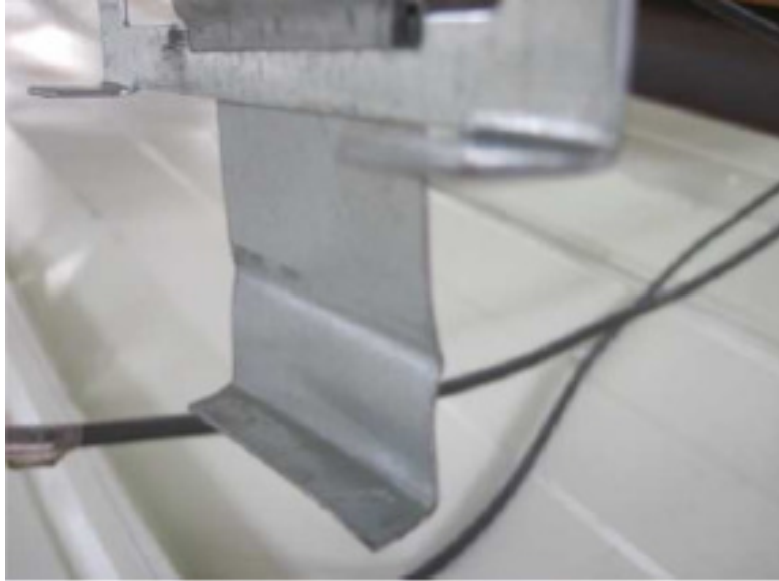
Figure 9: Straightened fastening clip after failure of fastening system (Song, Chen, & Zhang, 2010)
