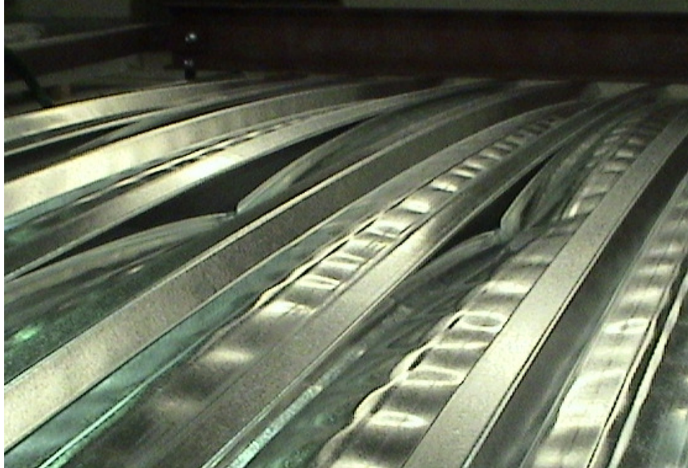
Figure 55: Local buckling at the fastening point indicated in red
