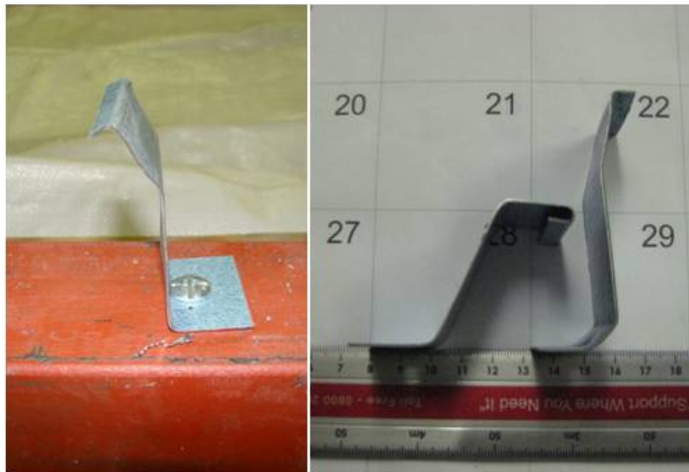
Figure 68: Fastening system failure due to cleat bending open
