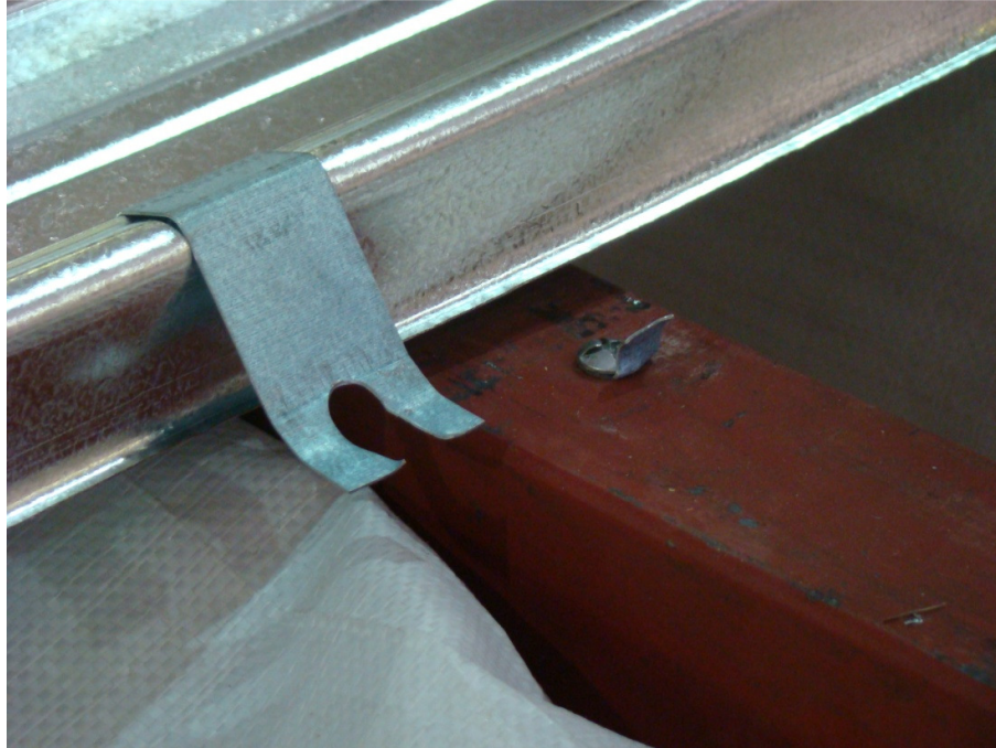
Figure 67: Fastening system failure due to tear-out
