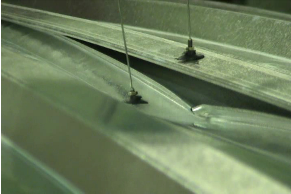
Figure 66: Local buckling in the male lip of the Craft-Lock sheeting system has occurred at 2.09kPa (as in Figure 64)
