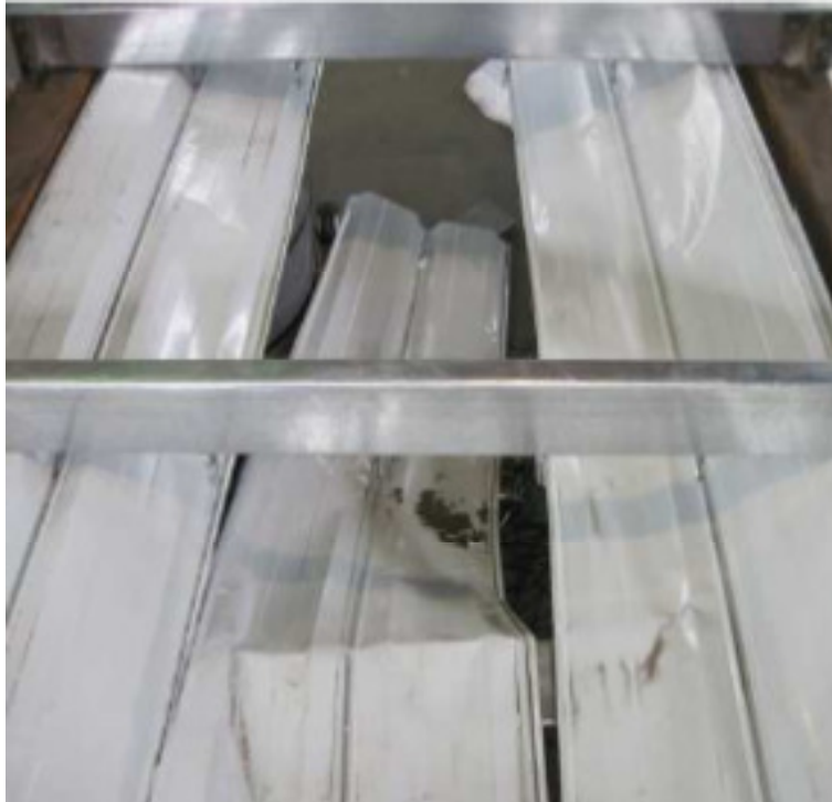
Figure 7: Ultimate failure in the sheeting system (Song, Chen, & Zhang, 2010)
