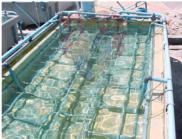
Figure 2.10 Pipe layout of grid and airlifts, the collection lines on the top of the tank and the two hydrocyclone filters at the top end.
