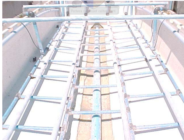
Figure 2.9 Pipe layout for the grid design and airlift pumps, drain and airlines.
