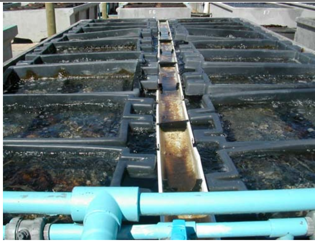
Figure 2.11 Modified PVC guttering with baffles, in the centre of the tank between the abalone baskets.
