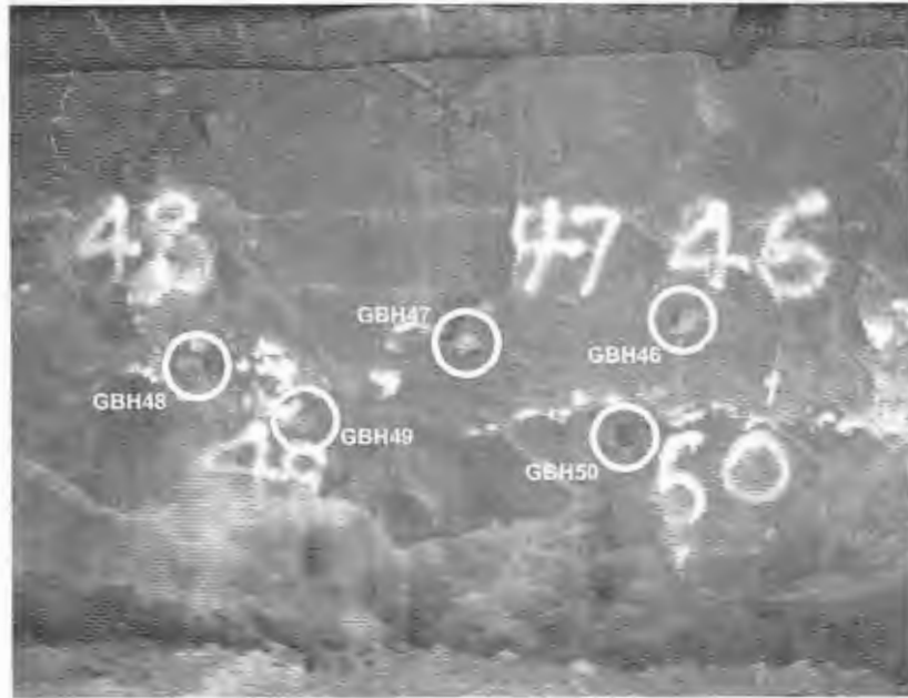
Figure F-2: GBH46 - GBH50 borehole collars at 13 Level West Haulage, Bleskop.
