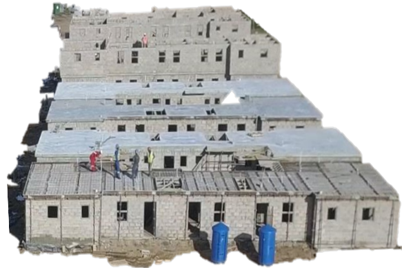
Figure 41. Hybrid Suspended Slabs Packed (Monitoring Image 4)
