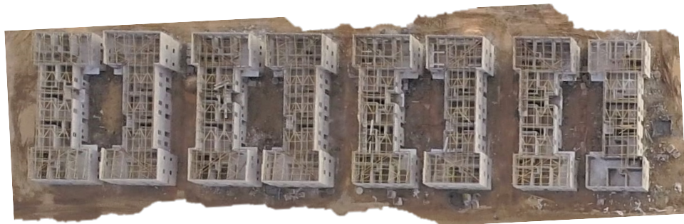
Figure 42. Hybrid Suspended Slabs Cast and First Floor Blockwork Commencing (Monitoring Image 5)
