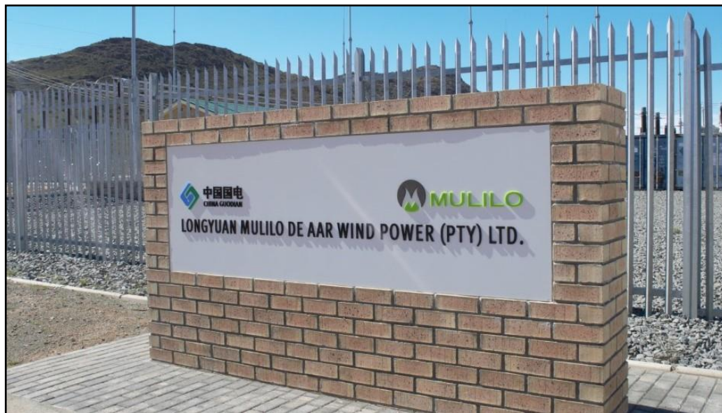
Figure 8.1: Longyuan Mulilo De Aar Wind Power substation entrance, 2018
