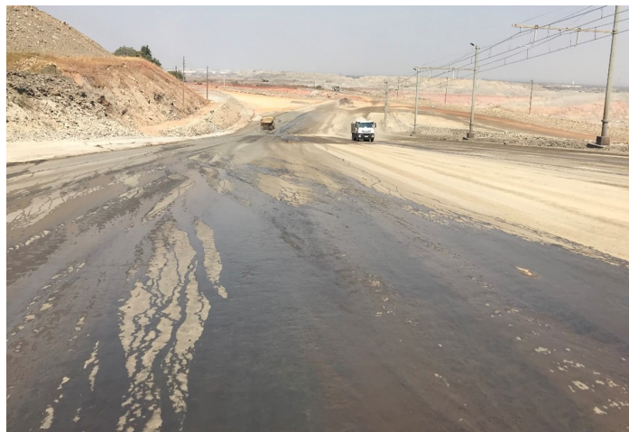
Figure 2.13: Dust suppressant running off upon application
